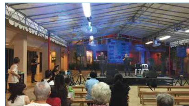
The open courtyard space of Kallang CC can accommodate a temporary shelter when needed as well as flexible stage and seating arrangements.
