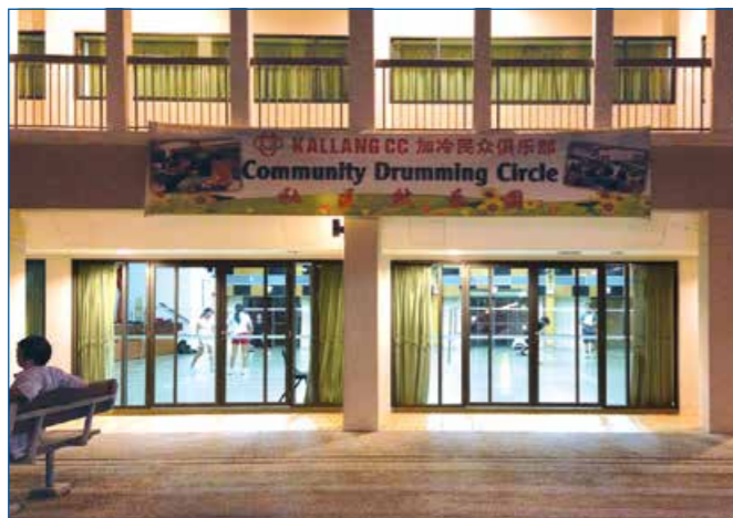
Glass façade of Kallang CC auditorium allows pedestrians passing by to see what is happening inside.
