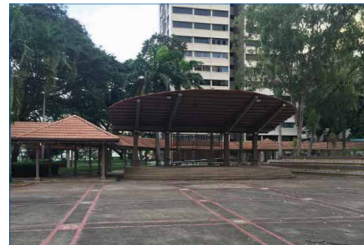
Bedok Neighbourhood Amphitheatre behind Block 35 Chai Chee Avenue
